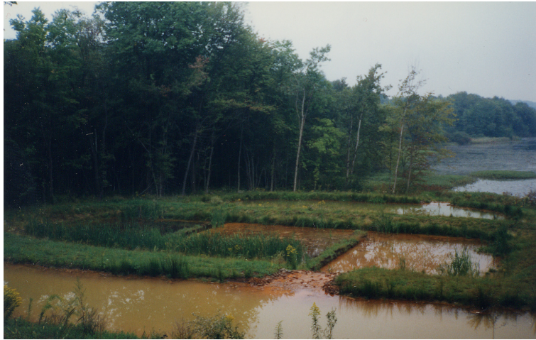
Figure 4. Constructed wetlands to treat acid mine drainage, Butler County, Pennsylvania. (Photograph by Jim Taylor.)
