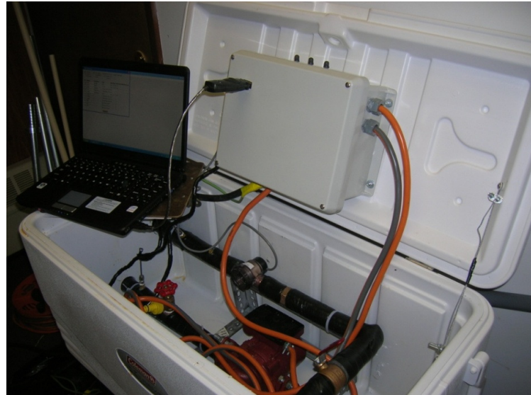
Figure 6 Test box with Computer connected to data logger
